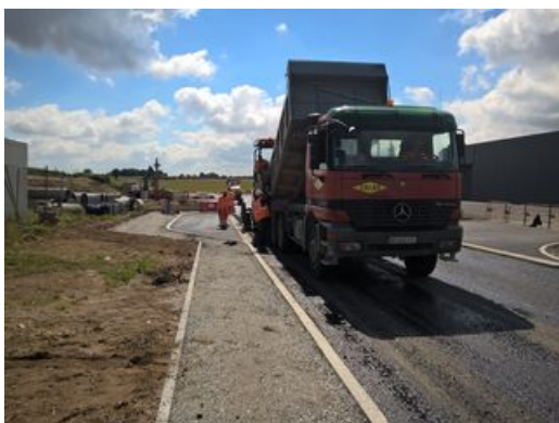
Travaux, Saint-Hilaire-de-Clisson, Site Aggloh, Site Habiter 26/07/2017
