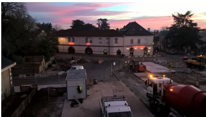
Travaux, Site Transports, Site Habiter 06/02/2017
