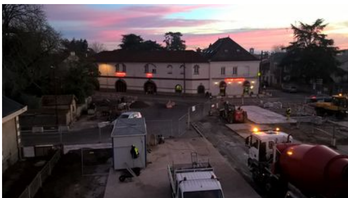
Travaux, Site Transports, Site Habiter 06/02/2017
